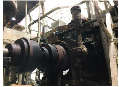
**APPLICATION DETAILS:** 377 HP @ 180 RPM **COUPLING INSTALLED:** T8 1018 Carbon Steel Floating Shaft with our corrosion resistant Melonite™ Flex Hub and Drive Ring. Torque Rating 262,600C/ 350,480P with Yellow HD Insert with Temp Range (-60/250)
